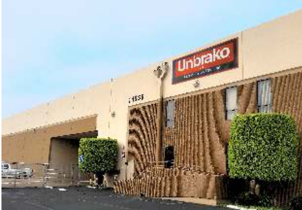
West Coast Distribution Center
